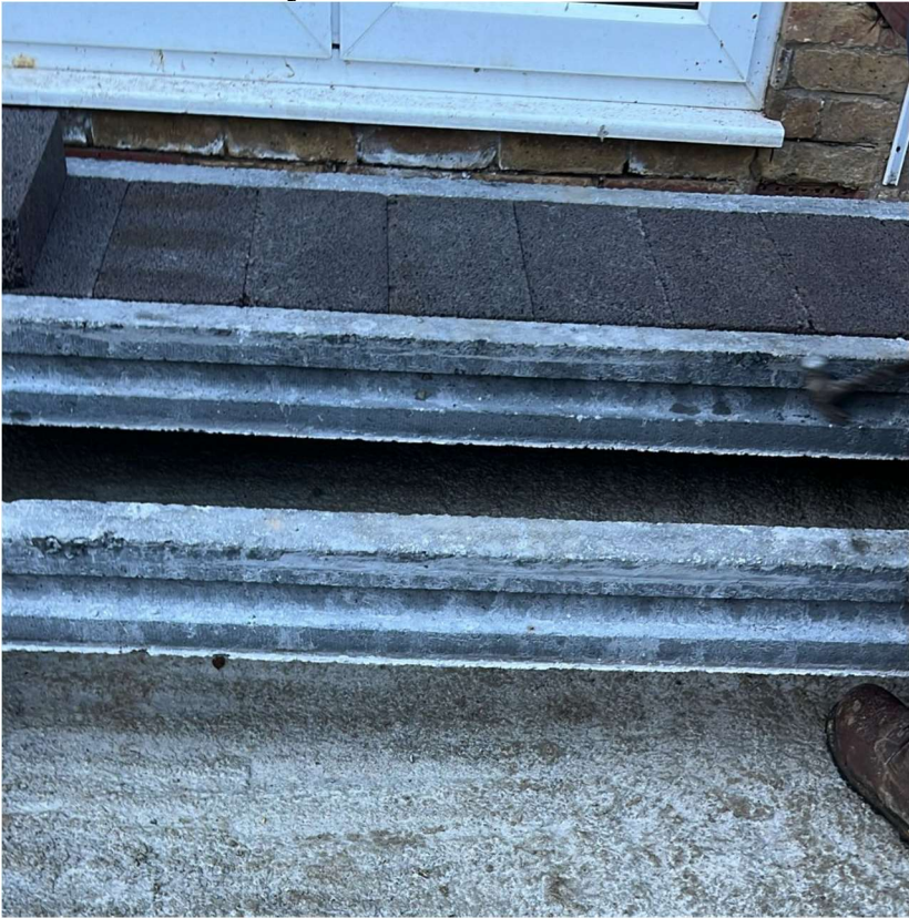
Fig 1 Starting to lay the block and beam
